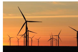
Figure 16. Traditional Wind Farm (courtesy of DOE)
